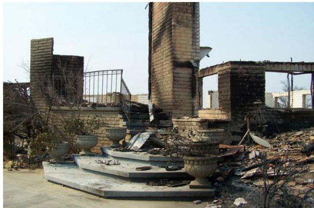
Jack and Mary Phillips' home after the fire. The Phillips decided to trade in this burned-down lot as a down payment on a new home.
